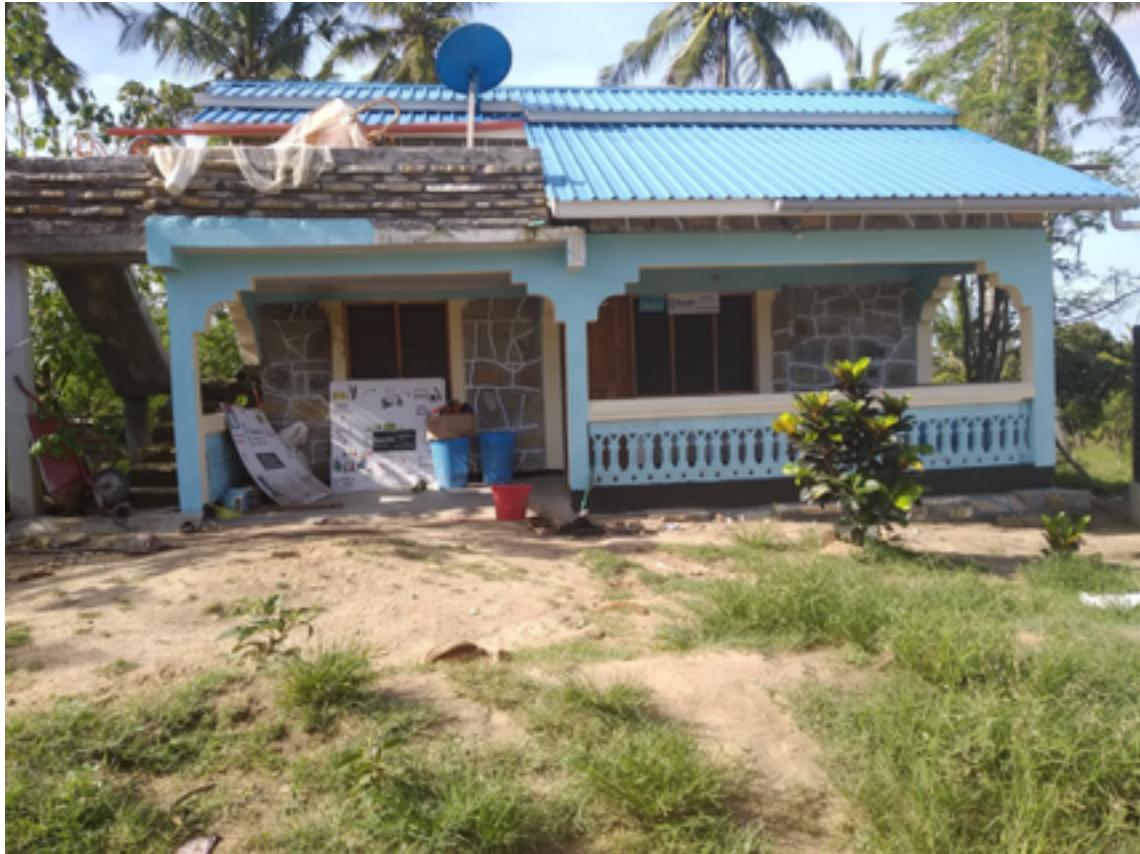
Picture 3.1 Shanga's Office. 2019 Photograph: Sowelu Avanzo
